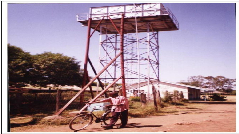
Plate 2: The tank and bore hole below which is the source of Ahero town piped water
